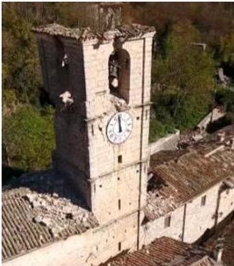
**Figure 2.** Belltower in Castelsantangelo, damaged by the earthquake in 2016 (confined tower)
