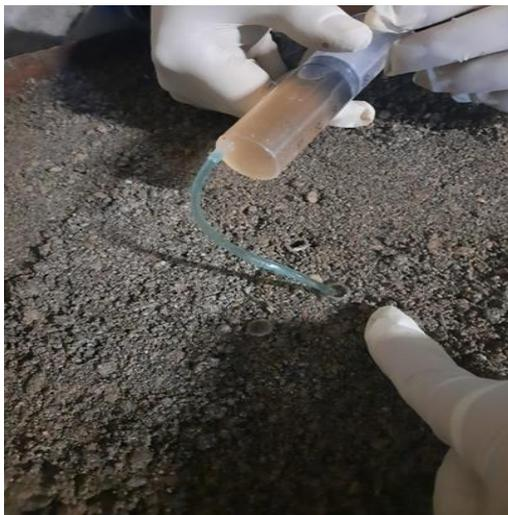
Figure 9. Bio-grout injection in micropile
