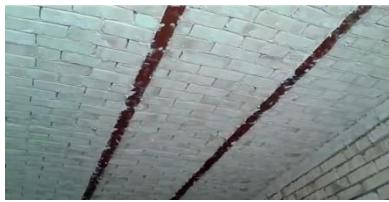
**Figure 1.** Brick slab after construction
