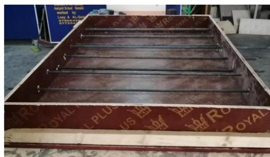
Figure 3. Preparing the CCB for light weight aggregate
