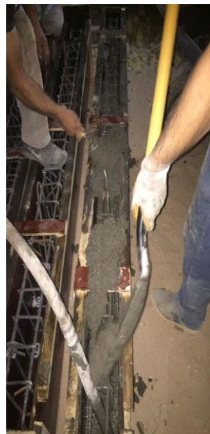
(b) Casting & vibrator
