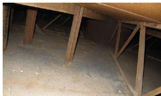
Figure 4. Detail of trusses and rafters of the roof
