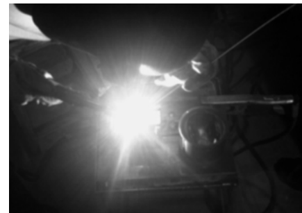
Figure 4. Capping the hole by Argon gas welding
