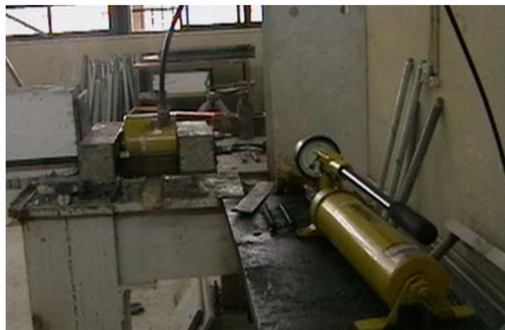
Figure 4. Post-tensioning using hydraulic jack
