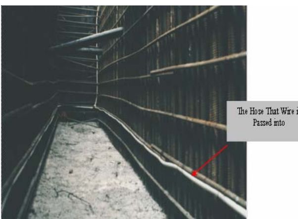
Figure 5. Passing the wire into the hose in RC wall.
