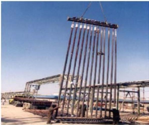
**Figure 4.** A view of exchange of the damaged tubes and the catalyst.
