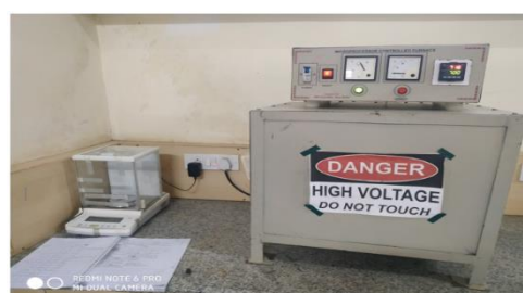
Figure 2. The silicon carbide tube furnace used for high temperature corrosion studies
