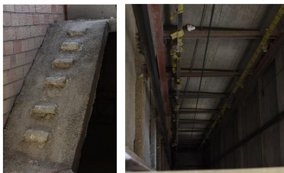
Figure 3. Under-construction condition of the building's stairway and elevator
