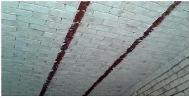
**Figure 1.** Brick slab after construction
