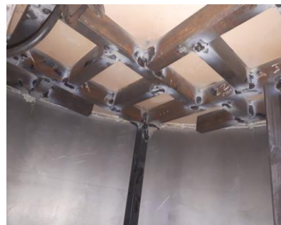
Figure 4. Steel grid in the roof of the tank
