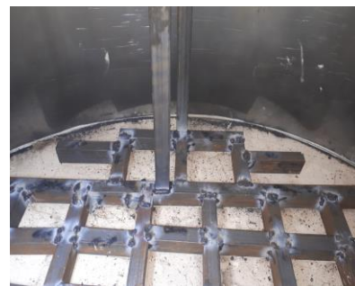
Figure 3. Steel grid at the bottom of the tank
