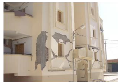
Figure 11. View of building B1
