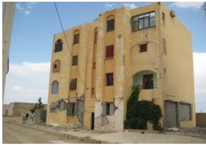
Figure 12. View of building B2
