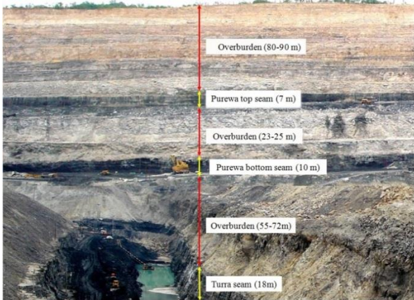
Figure 6. A typical cross sectional view of mine under study
