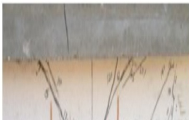
Figure 3. Cracking and failure pattern of beam B2.5-B
