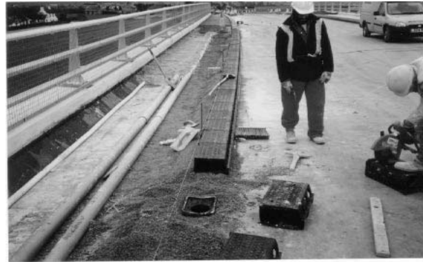
Figure 2 A construction view of CIS Bridgeflow II units.
