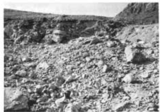
Figure 5. A typical good explosion where more than 90% of blasted rocks had less than one square meter dimensions.
