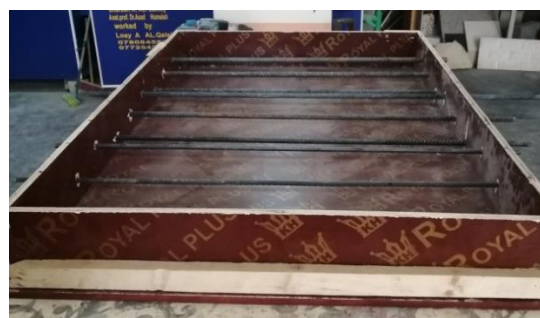
Figure 3. Preparing the CCB for light weight aggregate
