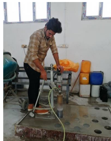
Figure 4. Concrete core drilling of LWC slab
