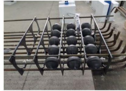
Figure 4. Preparation of the molded specimen and placing the reinforcement
