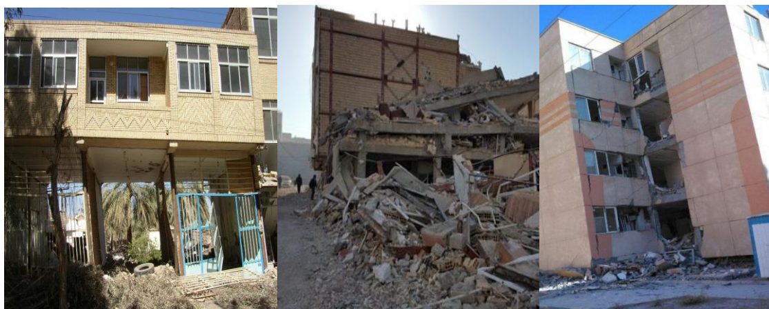
Figure 1. Damages caused by soft-story irregularity in Kermanshah Earthquake, 2017
