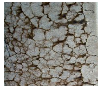
Figure 2. View of alkali silica reaction phenomenon
