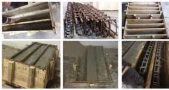
Figure 4. Preparation of original beams
