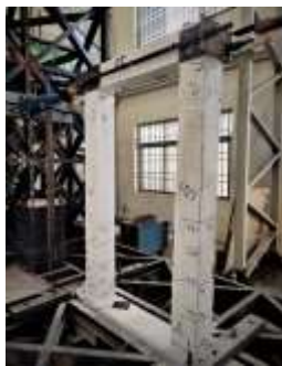
Figure 11. Cracks in CC frame after cyclic load
