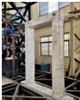
Figure 12. Cracks in CSC frame after cyclic load
