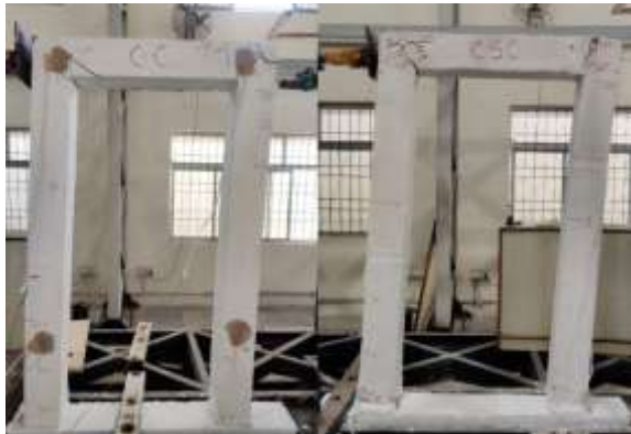
Figure 10. Cracks in CC and CSC frames after lateral load
