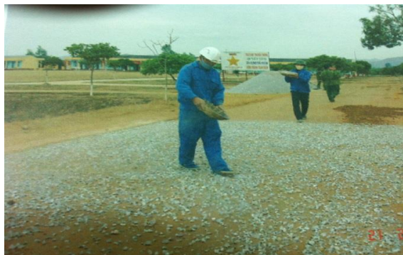
Figure 21. Stapling stones to create adhesion
