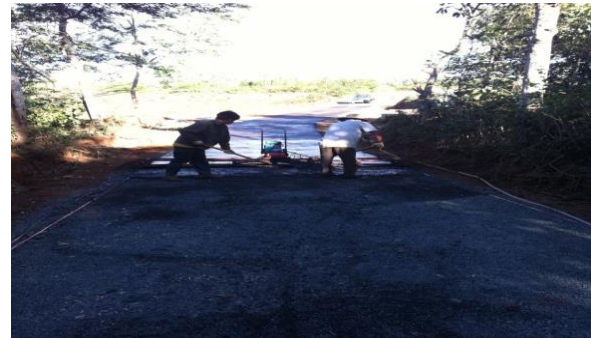
Figure 22. Making the asphalt mortar layer
