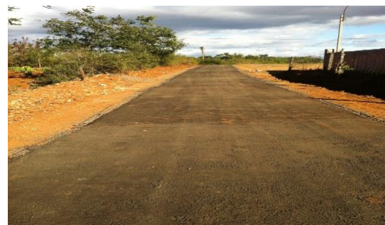
Figure 13. The road after covering the surface layer
