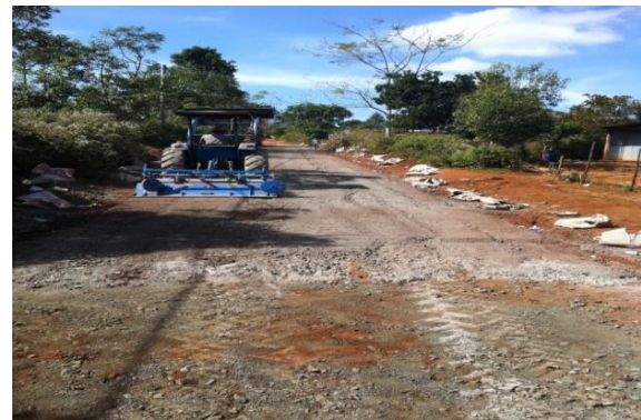
Figure 17. Milling machine to mix cement CB40 with basalt
