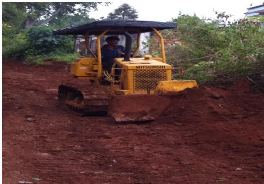
Figure 14. Bulldozer leveling the ground
