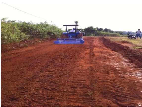
Figure 15. Plowing machine stirring the soil
