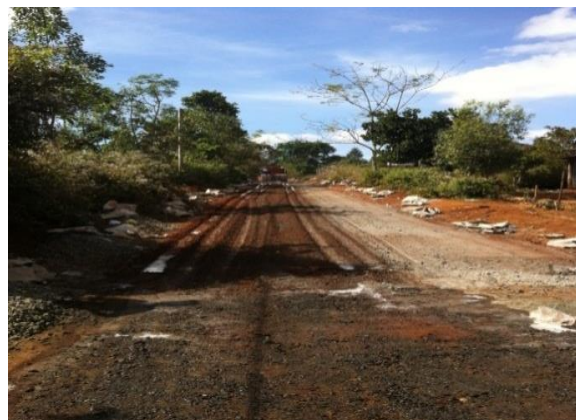
Figure 18. Watering with additive DZ33 added
