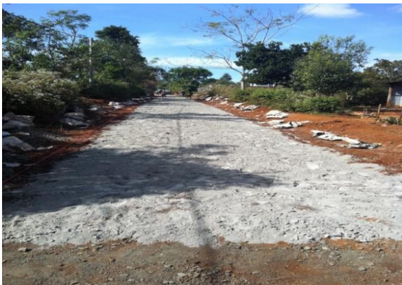
Figure 16. Spreading cement PCB40
