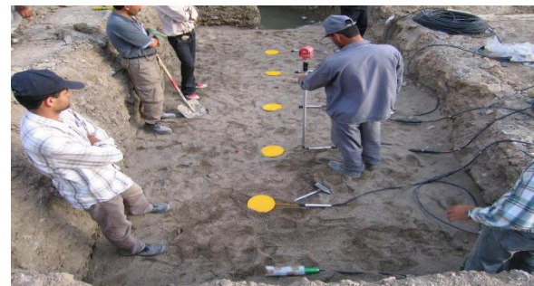
Figure 2. Installation of Instrumentations
