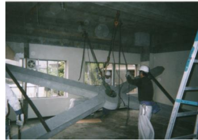
Figure 2. Erection of the brace
