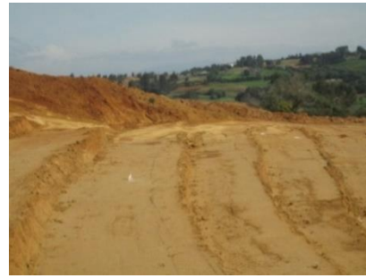
Figure 2. Site of embankment 3119
