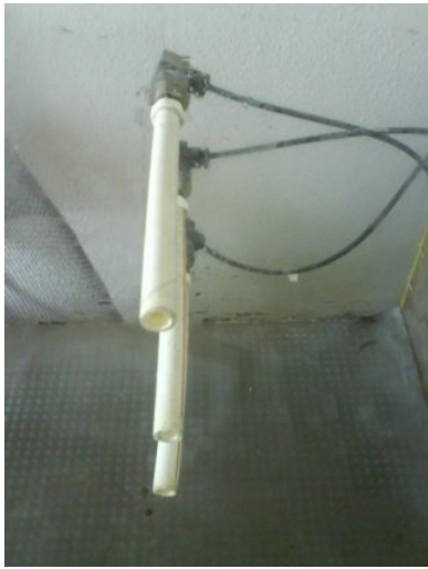
Figure 8. Installing tank accessories
