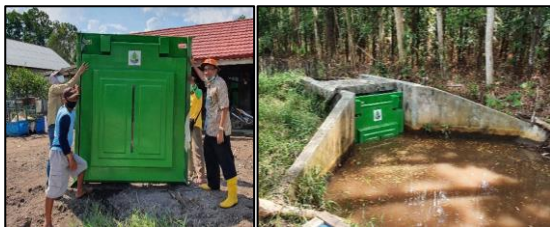
Figure 2. Example of using GFRP flap gates in swamp irrigation channels in Central Kalimantan Province, Indonesia
