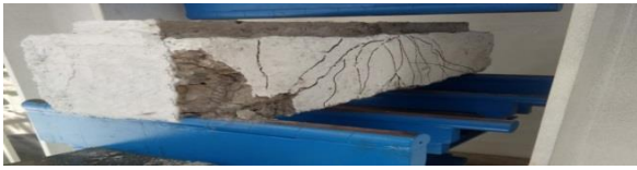
Figure 17. Beam failure and crack distribution of RCJ6 beam
