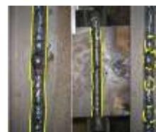
Figure 2. Welded area after welding operation
