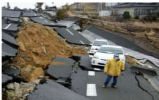
Figure 1. The earthquakes on the structures built on collapsing soils
