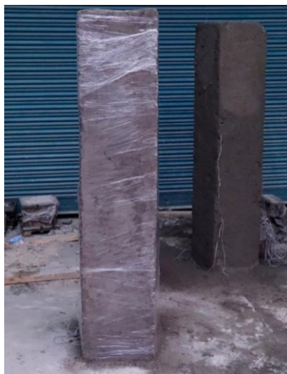
Figure 4. Plastic curing for column CSAF
