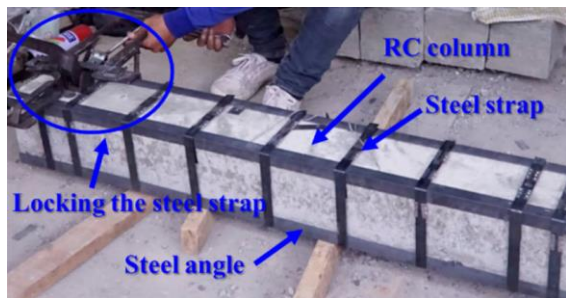
Figure 3. Strengthened column
