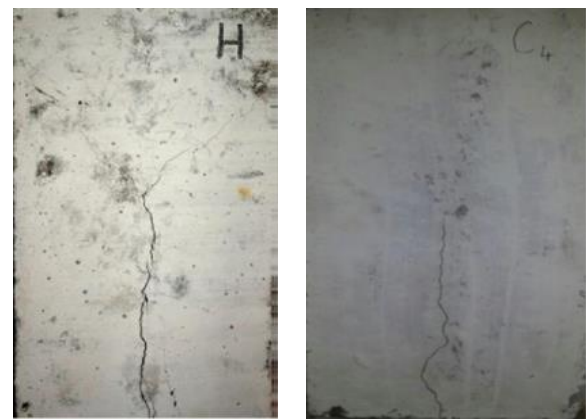
Figure 12. Crack pattern in beam-end specimens
